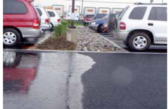
Non-Porous vs. Porous Asphalt
